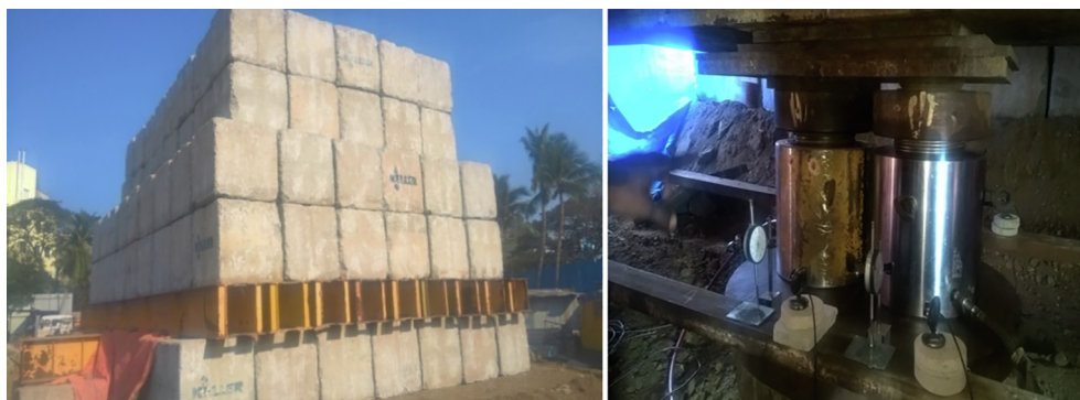
Fig. 3. Kentledge arrangements and loading/unloading hydraulic jack.
