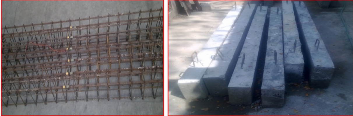
Fig. 2. Reinforcement cage and Casted beam.
